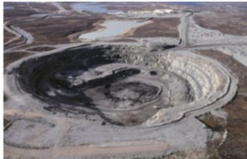
*Excavation of a pipe is carried out in a way that creates a spiral roadway along the perimeter of the mine. As the pit gets deeper, benches are cut in the surrounding rock to keep the walls from collapsing.*
